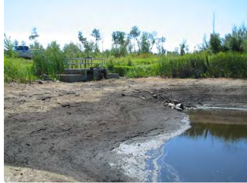
Dry pool – gate malfunction
