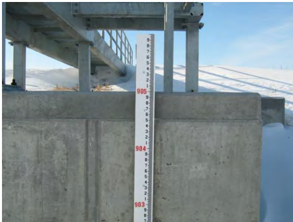
Typical staff gage at structure
