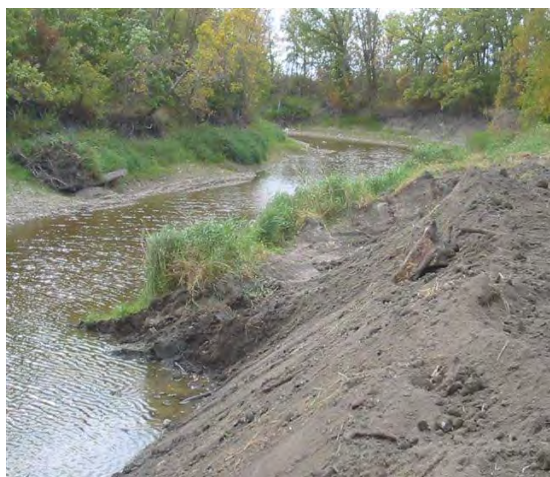
Downstream end of sediment bar
