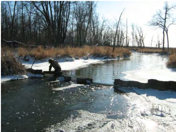
Installing stoplogs at sheet pile dam
