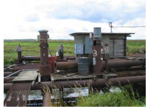
Typical pumping station
