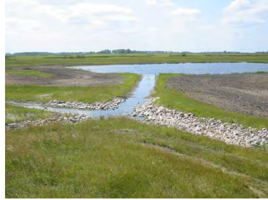
Interior ditches and borrow area
