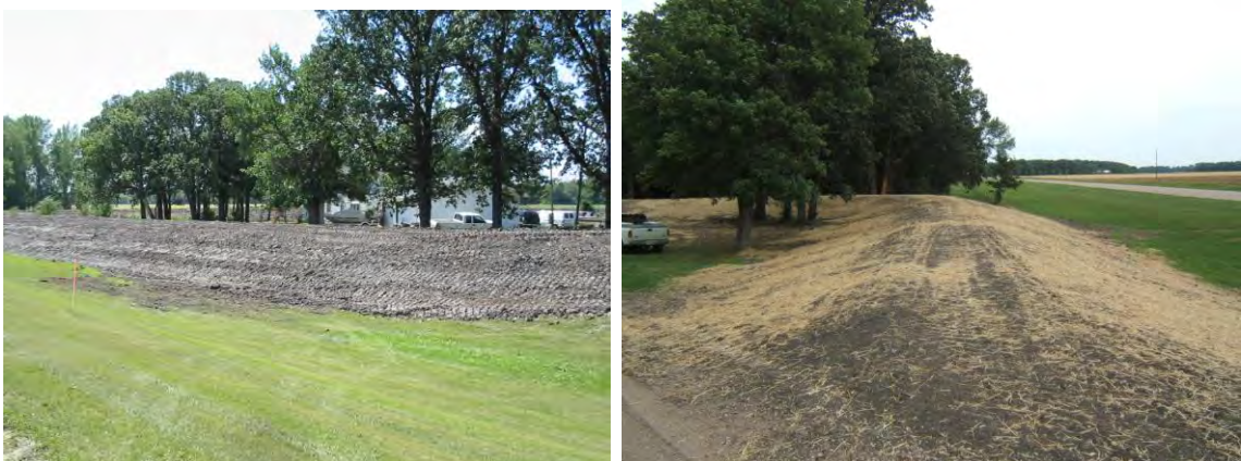
Shannon Schauer ring dike construction located in Section 27, Esther Township, Polk County. Near the Red River of the North.
