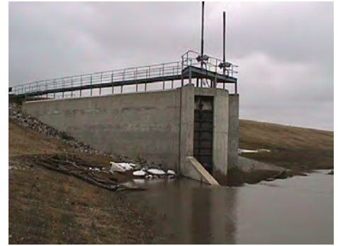
Principal outlet structure hydraulic gate operation
