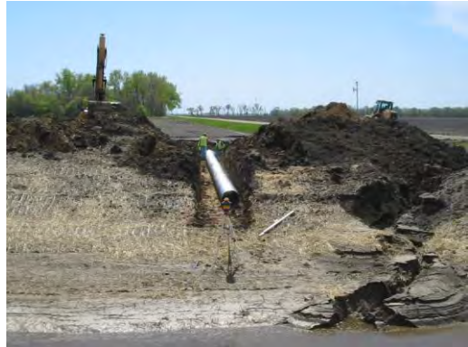
Installation of field drainage culvert
