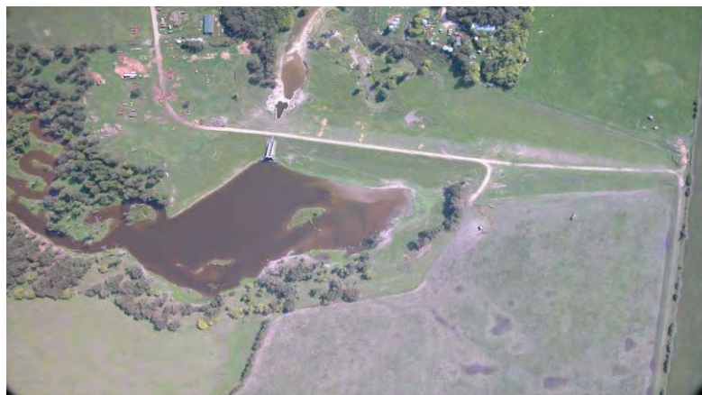
Aerial view of Schirrick Dam looking south
