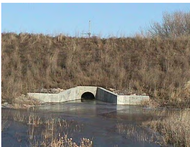
Principal outlet structure
