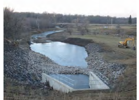
Looking downstream from outlet structure
