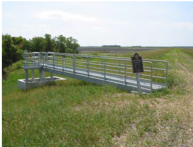
Principal Outlet Structure
