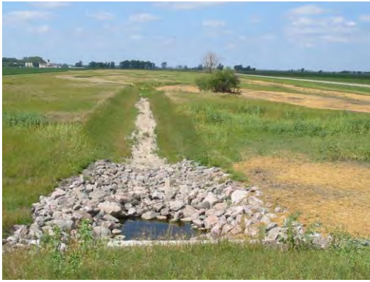
Principal Outlet structure looking west
