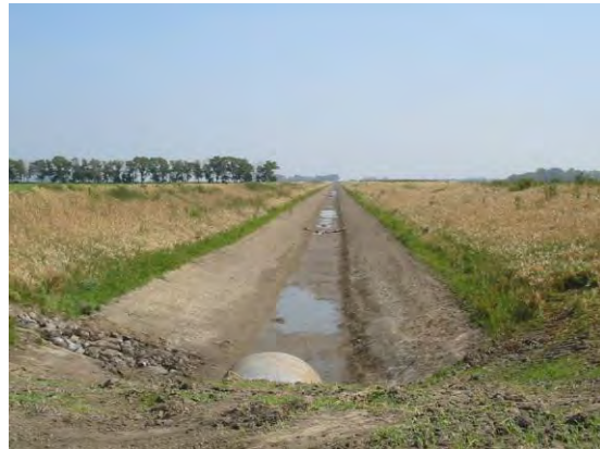
Completed ditch section
