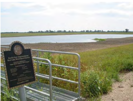
Looking southeast from outlet structure
