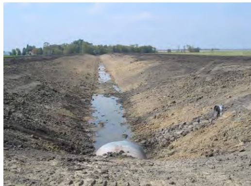
Recent excavation near outlet of ditch
