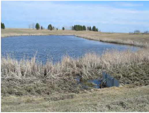
Thibert Dam, Red Lake County
