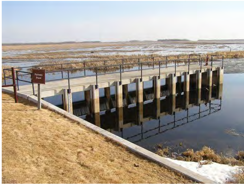
Stoplog Outlet Structure
