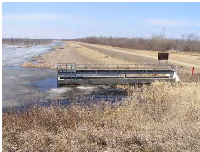
North Pool - Gated Principal Outlet Structure
