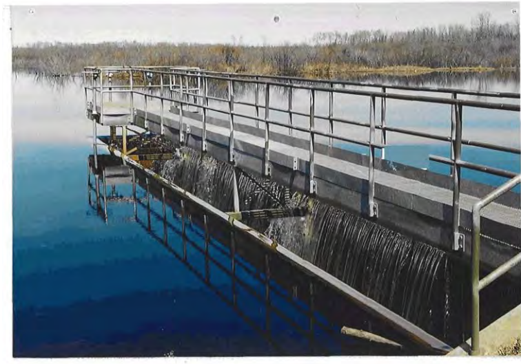
South Pool - Gated Principal Outlet Structure
