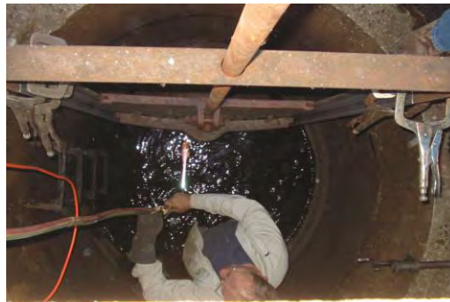
Gate repair inside structure
