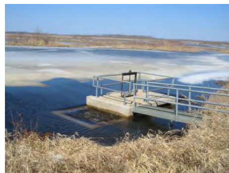
Gated Principal Outlet Structure
