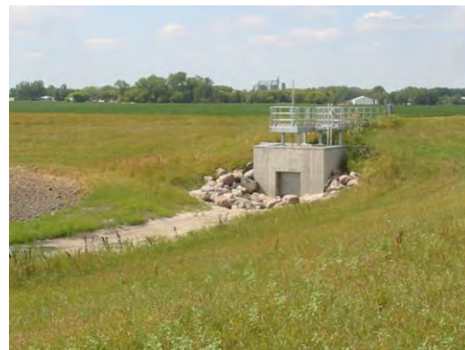
Principal Outlet Structure
